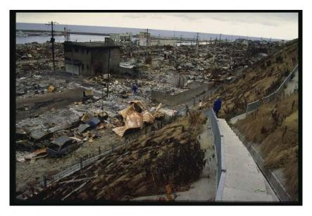
1993 Hokkaido earthquake and tsunami: Aonae, Okushiri Island, looking southeast. Structures in the foreground were damaged by fires fueled by above-ground kerosene and propane tanks following the tsunami. The concrete steps provided a means of escape for some residents following the strong earthquake<sup>2</sup>
